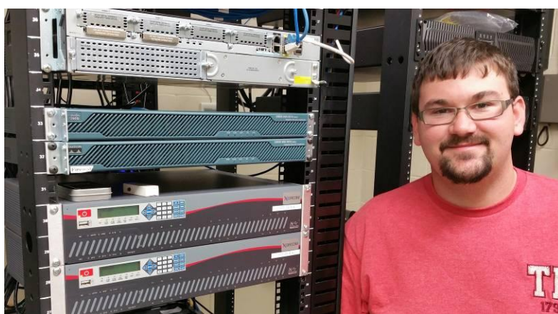
Chris Barnett of the Crossville IT team, next to the Xorcom IP-PBX servers, which are part of the TwinStar configuration for high availability.
